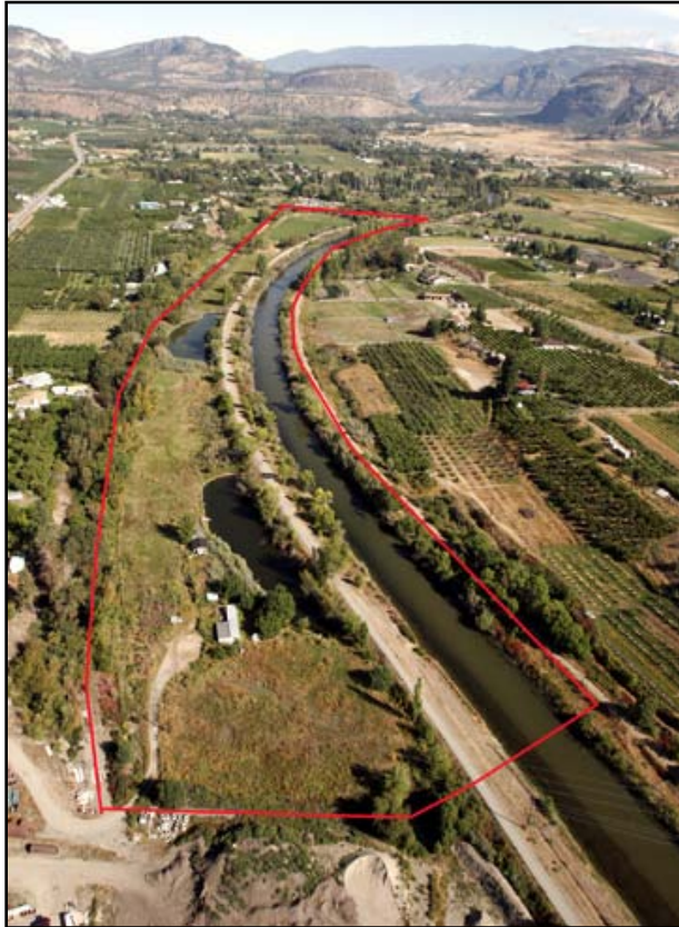
Figure 1: Phase I Okanagan River - Illustrating Pre-restoration Conditions
