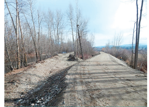
Removal of the old dike (left) and construction of the new dike (right) were scheduled during low-water times to prevent ecological damage.
